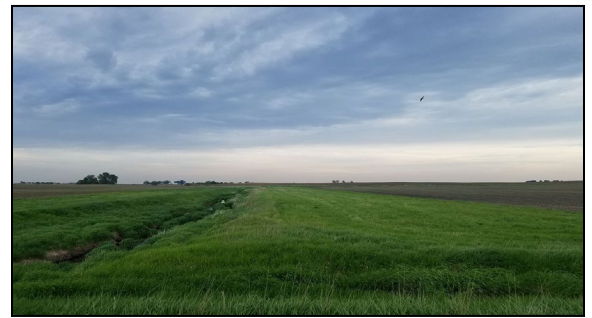
Filter strip in a field. Photo courtesy of Dallas SWCD.
